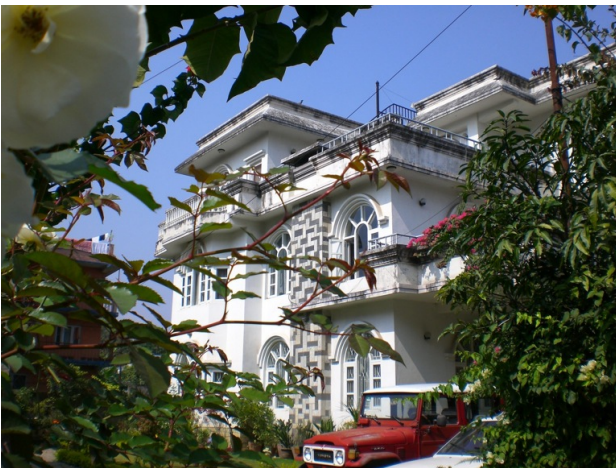
The NRC office at Baluwatar
