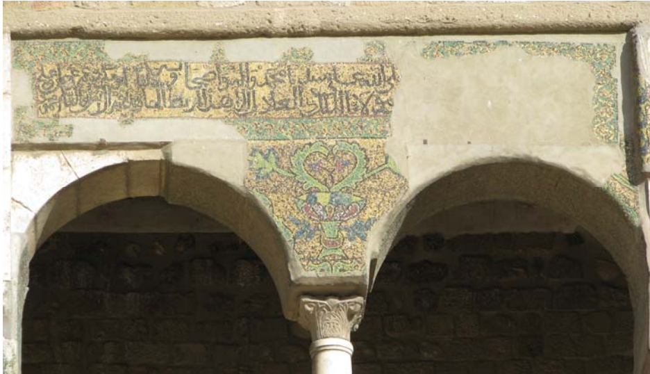
Fig. 05 – Damascus, Umayyad mosque, mosaic inscription by Nur al-Din Mahmud, probably after the earthquakes (photo author).
